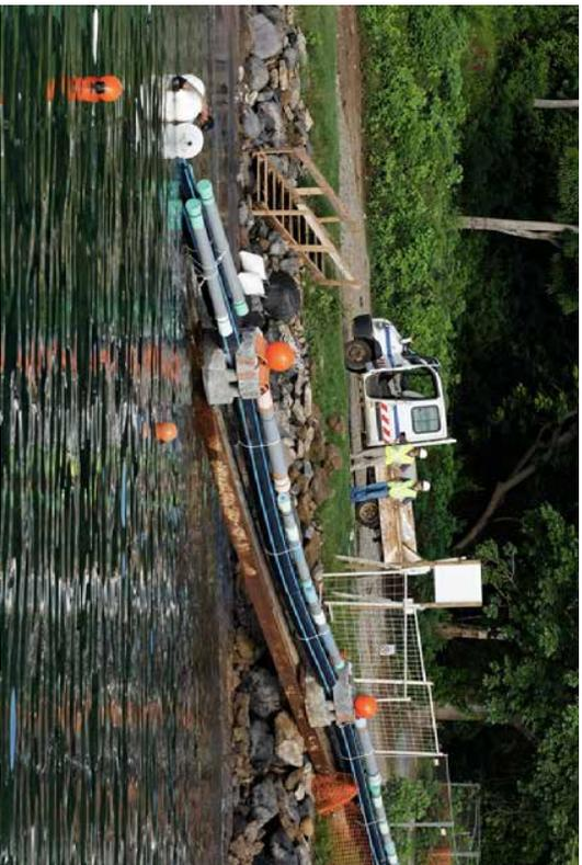
Figure 23: Installation work for eco-designed pipelines in Mayotte in 2009 (© L. Cadet)
