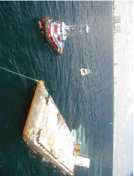
Figure 1: Submersion of artificial reefs made up of blocks of calcareous rocks in compensation for the degradation of coral reefs in Florida (© S. Ploch)
